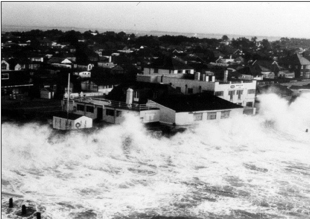
Plate 2: Wave overtopping adjacent to Creek Road car park, pre Beach Replenishment 1985
