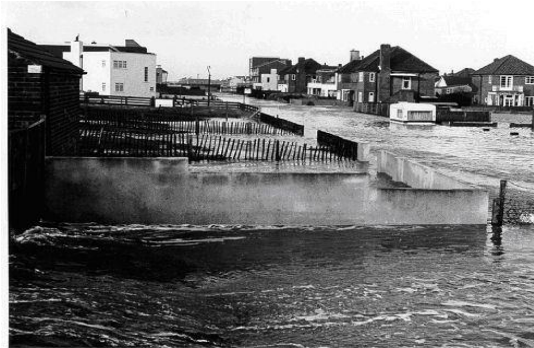
Plate 1: Storm damage to properties behind the seawall, December 1978
