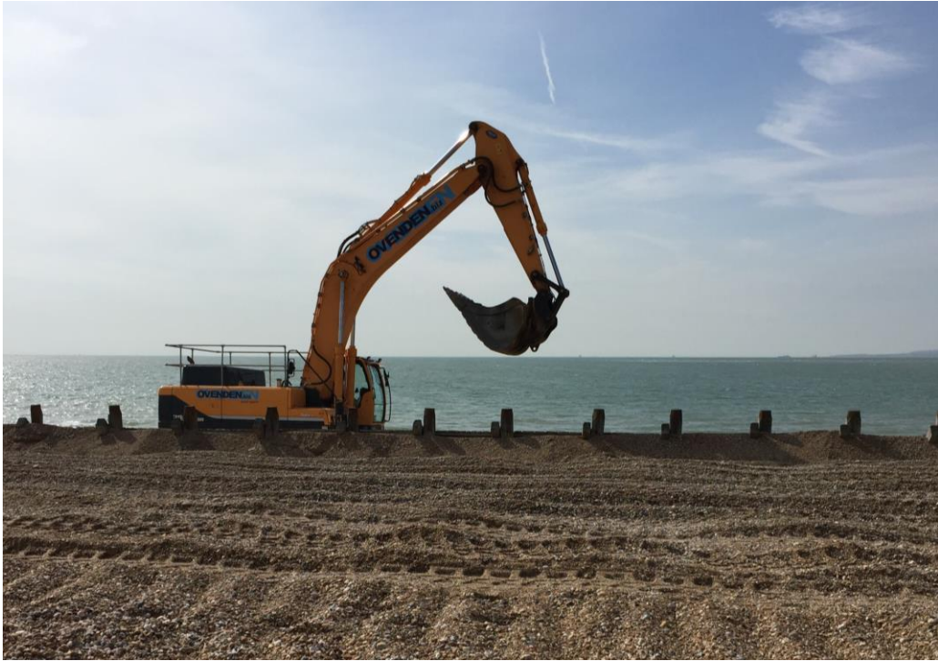
Plate 3: An excavator on site at Hayling
